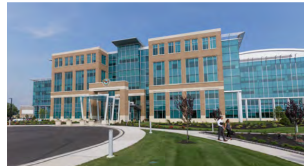
Two recent additions to our portfolio of green buildings are the LEED-Gold certified Pratt & Whitney engineering & technology center (top) and the United Technologies research center (bottom), both located in East Hartford, Connecticut.
